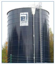
The interior of the 0.75 MG Depot Road Tank was resealed in 2017. The tank was originally constructed by Mid-Atlantic Storage Systems in 2002. The 45-feet diameter, 65-feet deep bolted steel tank provides water for average and peak day use and emergencies (such as power
