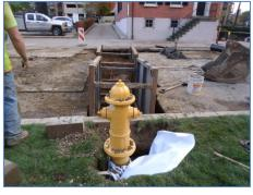
This project replaced 750-feet of 4-inch water main (installed in 1887) along East 2<sup>nd</sup> Street between French Street and Holland Street. The water main had experienced many recent breaks and was also undersized to accommodate the new UPMC Hamot Patient Care Tower project planned for 2018/2019. A new 12-inch ductile iron water main was installed by Chivers Construction Company. EWW staff designed and bid the project worked with UPMC Hamot to phase the work with
