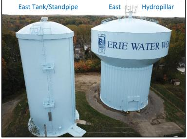
tank holds 800,000 gallons while the hydropillar contains 1,500,000 gallons of water. The interior and exterior were recoated in 2020 and new, continuously operated, mechanical mixing systems were installed in order to promote uniform water quality and to help control disinfection byproducts. Circulating water in storage facilities helps to keep chlorine levels uniform, to reduce water age in the distribution system, and to prevent thermal stratification year round.
