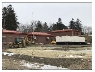
Improvements to the Cherry Street Pump Station are wrapping up. Work included eight new pumps, electrical upgrades, emergency power generators, and a sodium hypochlorite disinfection booster system. This critical station pumps water to over 40,000 people in portions of Erie, Harborcreek, Millcreek, Summit, and Wesleyville.
